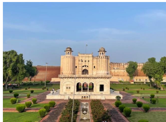
Figure 6: Hazuri Bagh Baradari now, without its upper level, having Alamgiri Gate in the background. Source: Department of Archeology, Govt. of Punjab
