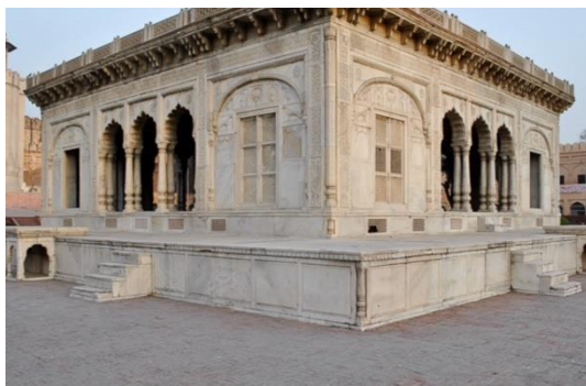
Figure 7: White marble baradari situated on three feet raised platform in the centre of Hazuri Bagh.
