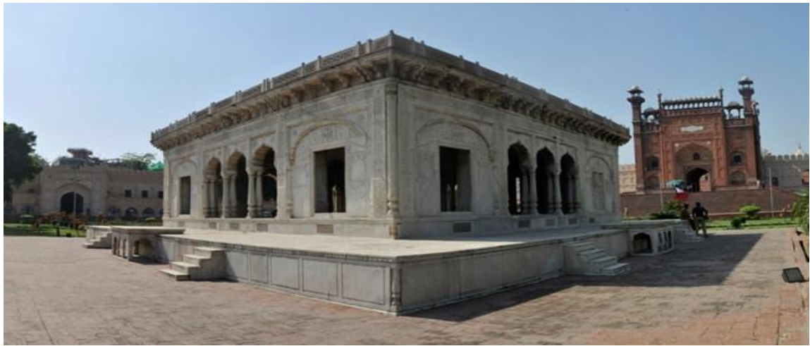
Figure 3: Hazuri Bagh Baradari, with the front façade of Badshahi Masque in the background (Source: Author)
