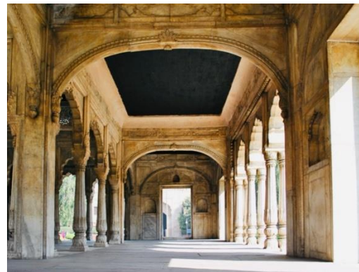
Figure 12: Ceiling of the side gallery renovated with deodar wood.
