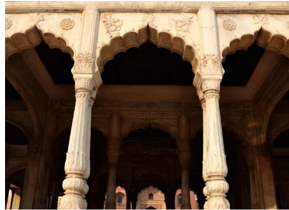
Figure 10: Interior view of the central chamber resting on twelve columns with scalloped arches.
